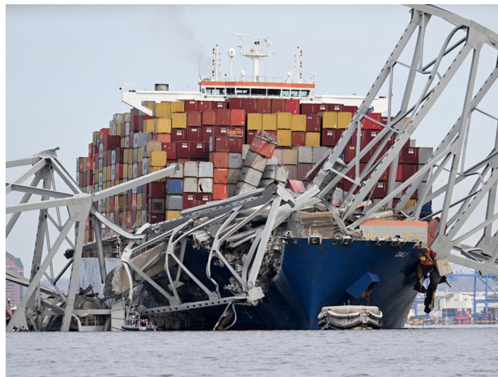
FSK Bridge Collapse (2024)
